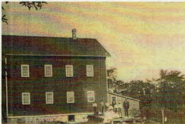
Messer Mayer Mill – 1912 ↑ Bridge, Mill Race, Flume & Engine Shed
